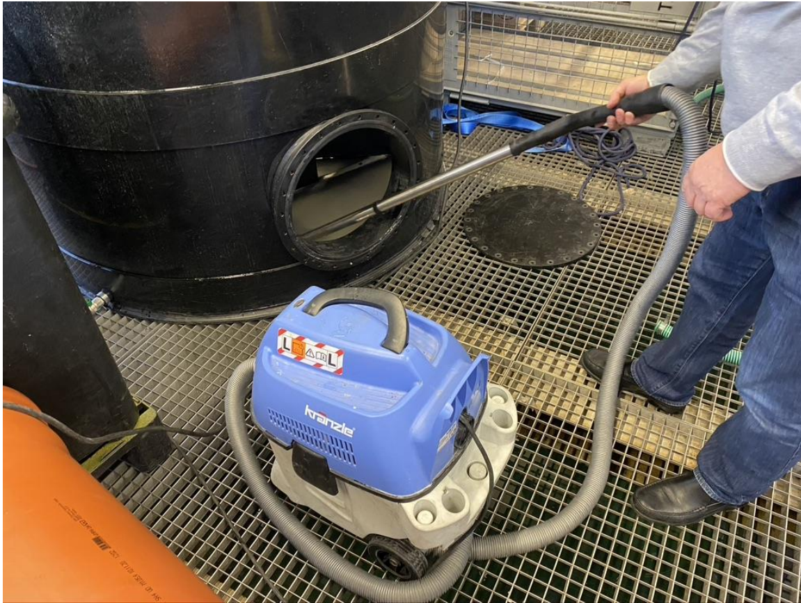
Figure 15 Captured Sediment Collected with Vacuum
